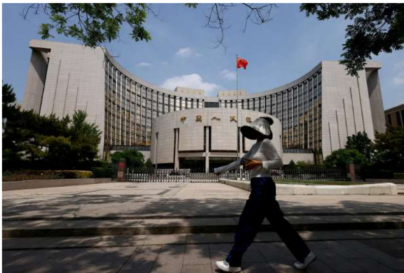
China built a $600 billion network of swap lines with central banks — offering liquidity while extending its reach beyond the dollar system. Tingshu Wang/Reuters
