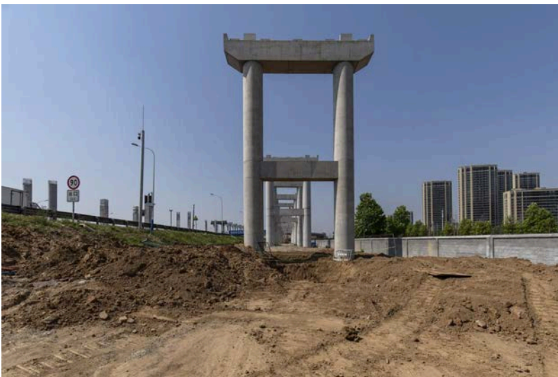
A highway under construction in Jinan, China. PHOTO: QILAI SHEN/BLOOMBERG NEWS
